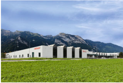
Heating system production in Sennwald
