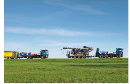
Borehole drilling by BauGrund Süd
